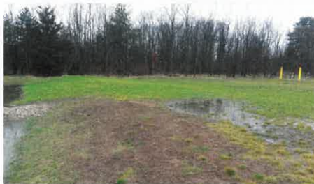
A flooded vegetative treatment area and the "background" monitoring well.
